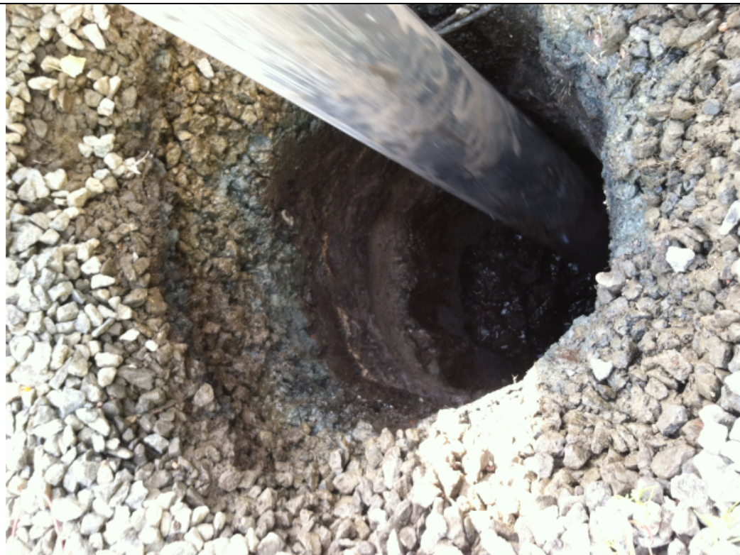
Photograph #2 – Vacuum soil extraction of an approximately 18-inch diameter hole.
