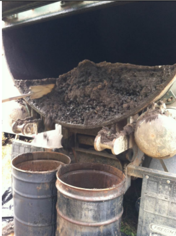
Photograph #5 – Transfer of wastes from the vacuum soil extraction unit into 55-gallon drums to facilitate off-site disposal.
