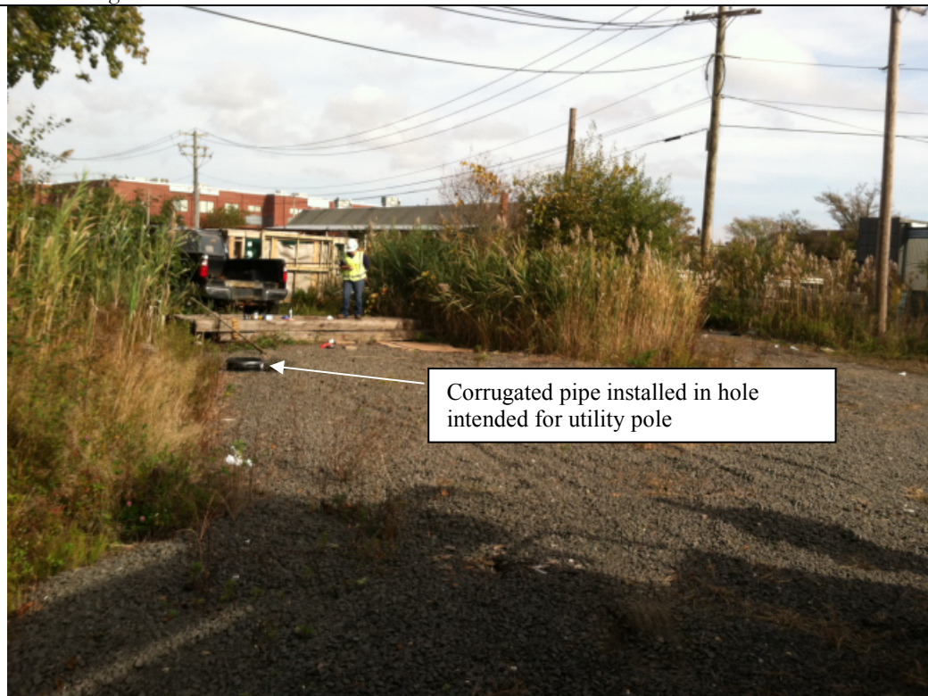
Photograph #4 – View of work area following vacuum soil extraction to target depth and subsequent installation of corrugated plastic pipe intended to stabilize sidewalls of hole.
