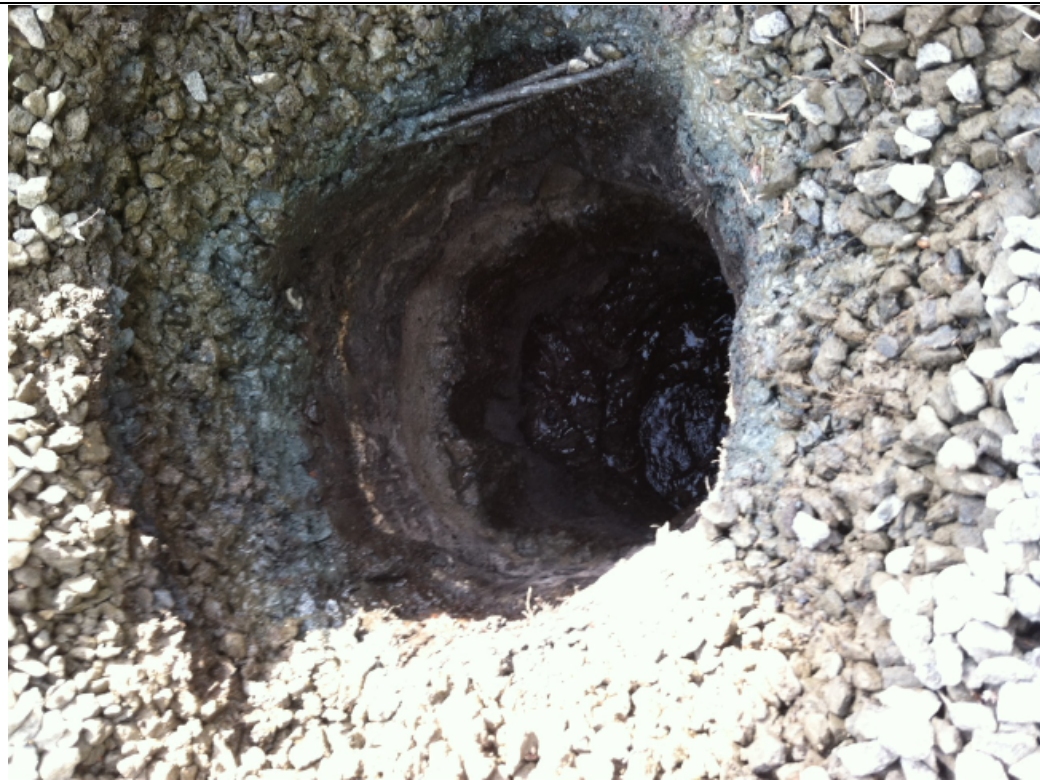
Photograph #3 – View of sidewalls and bottom of hole prior to utility pole installation. Note the groundwater seepage into the hole. Groundwater was encountered at a depth of approximately 2 feet below ground surface.
