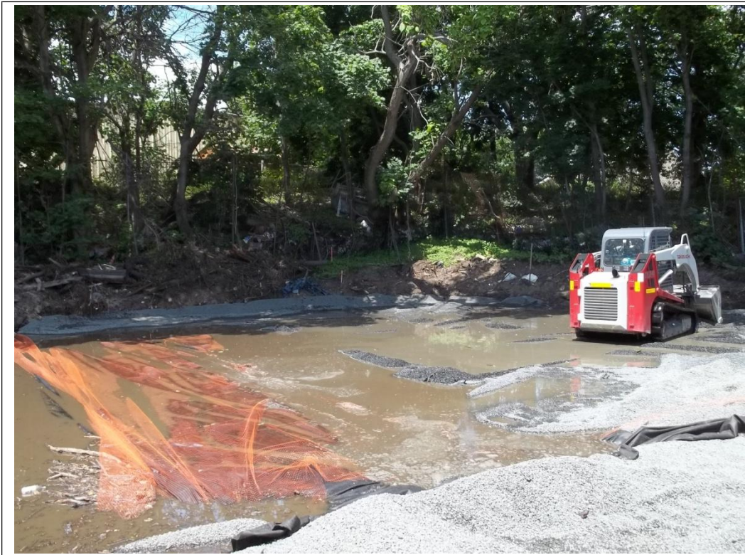
Photograph # 19: Date: 06/27/12 Photographer's Initials: DH Description: Placement of environmental cap in Northern portion of Utility Corridor
