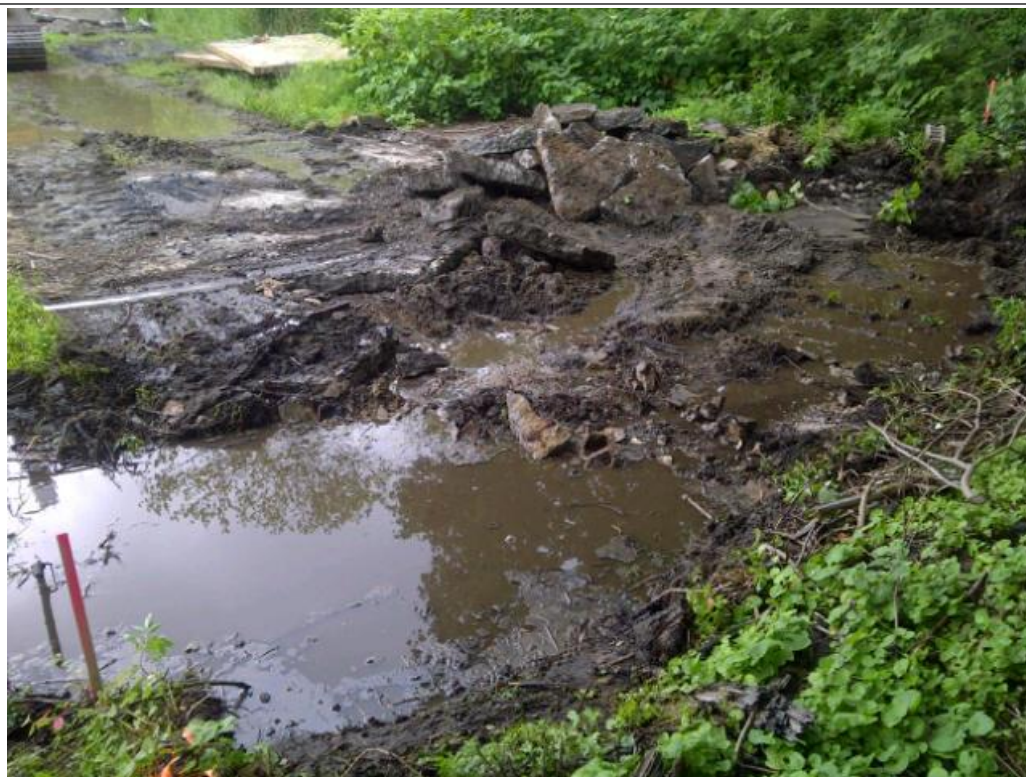
Photograph # 12: Date: 06/14/12 Photographer's Initials: DH Description: Removal of concrete pad over NAPL/Coal Tar-impacted area
