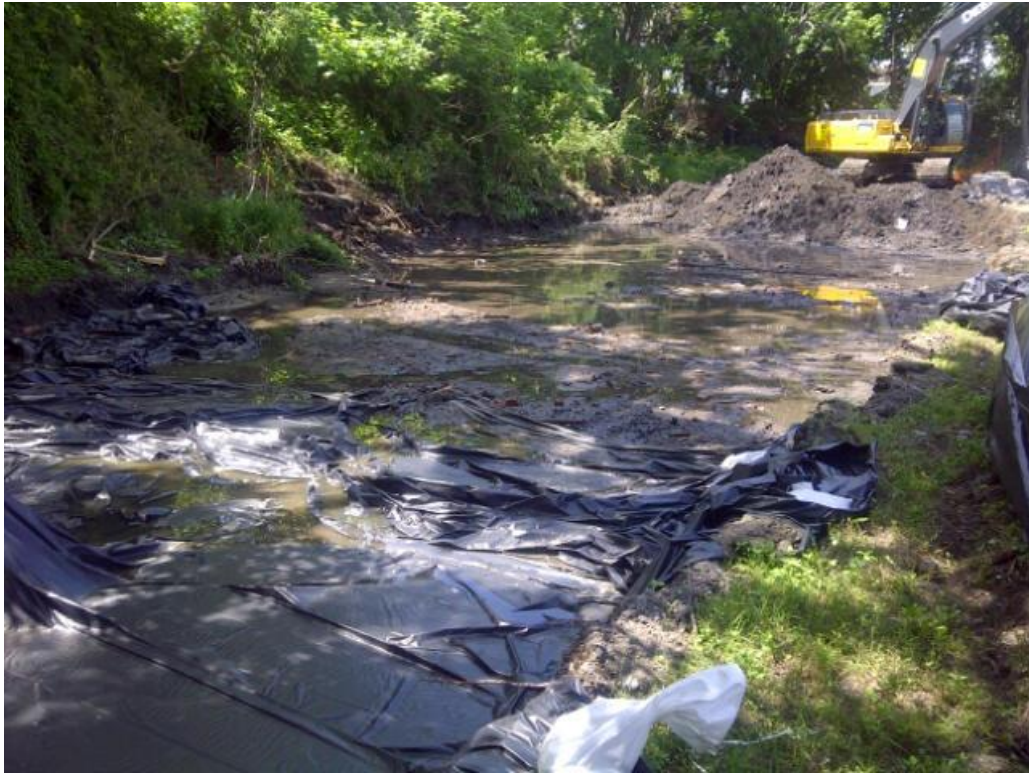
Photograph # 17: Date: 06/18/12 Photographer's Initials: DH Description: View looking North of Utility Corridor with geotextile placed on native soils (approximately 2 ft/bgs)
