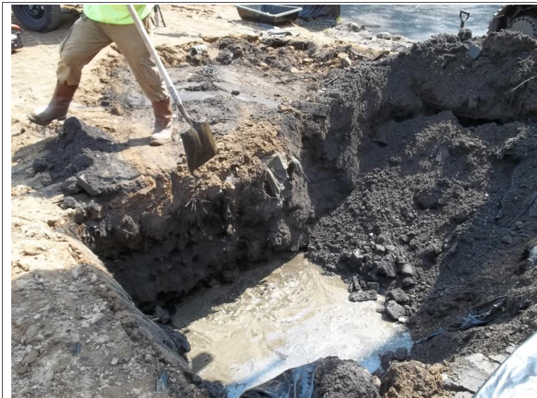
Photograph # 2: Date: 6/20/12 Photographer's Initials: DH Description: Test pitting to identify historical drip pot location
