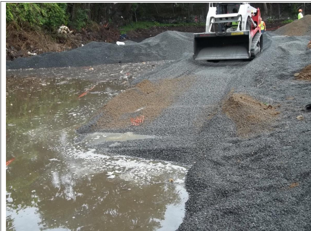
Photograph # 20: Date: 06/29/12 Photographer's Initials: DH Description: Placement of environmental cap
