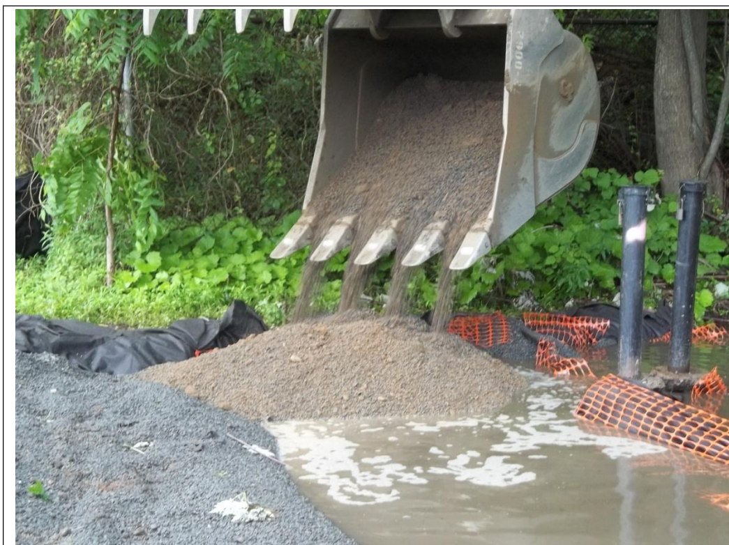
Photograph # 21: Date: 06/29/12 Photographer's Initials: DH Description: Placement of environmental cap around MW-7 well cluster
