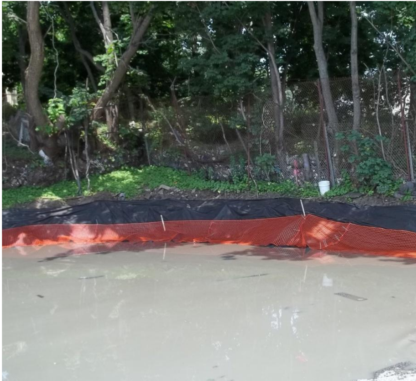
Photograph # 18: Date: 06/28/12 Photographer's Initials: DH Description: View of Northern embankment with geotextile and demarcation layers visible of Utility Corridor
