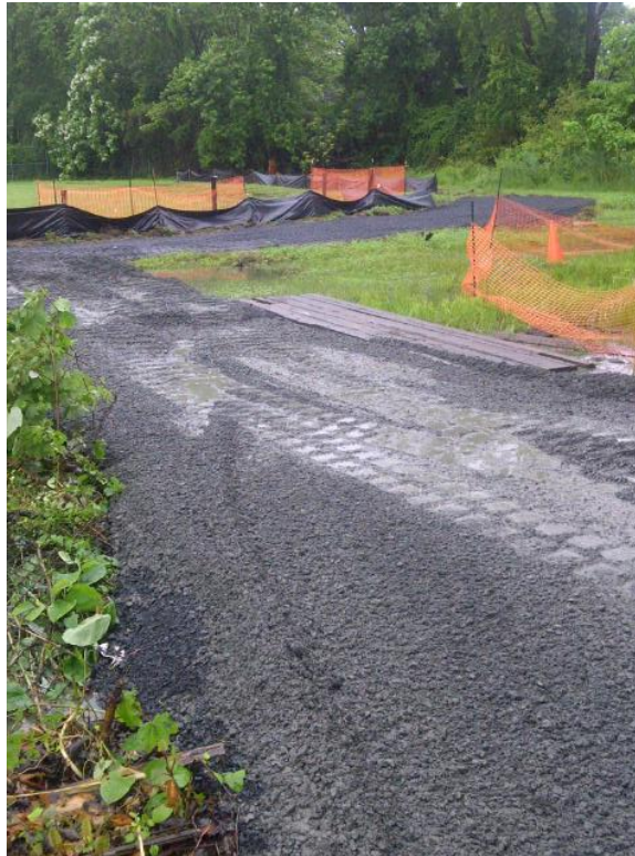
Photograph # 8: Date: 06/13/12 Photographer's Initials: DH Description: Completed on-site haul roads with construction mats visible
