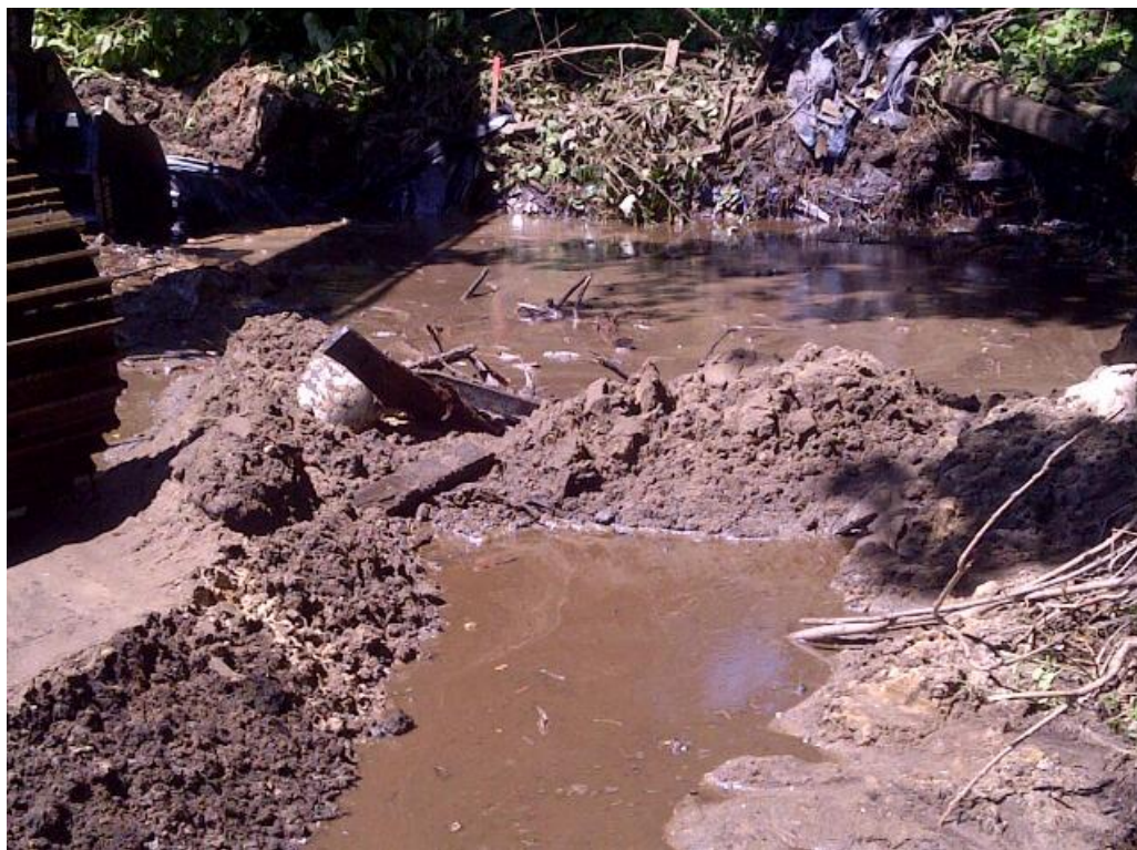
Photograph # 13: Date: 06/15/12 Photographer's Initials: DH Description: Excavation of soils in the northern portion of the Utility Corridor without dewatering
