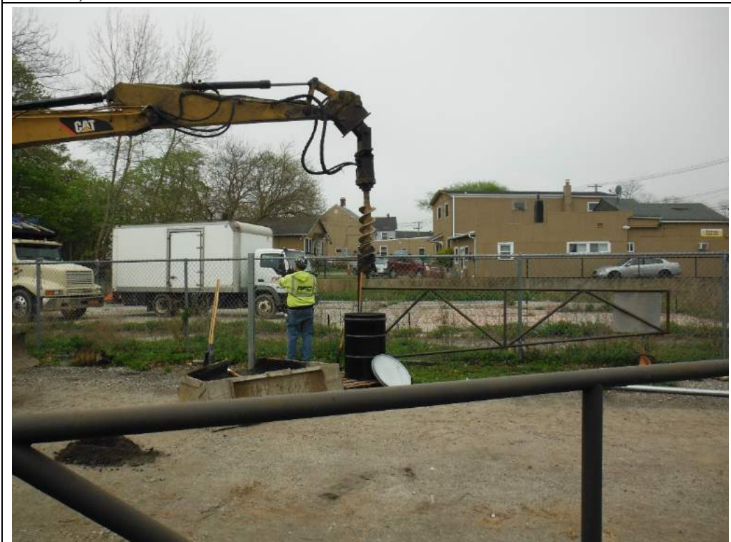
Photograph #6 – Contractors excavating gate post hole using a backhoe mounted auger, depositing soil into a 55-gallon drum (view looking west)
