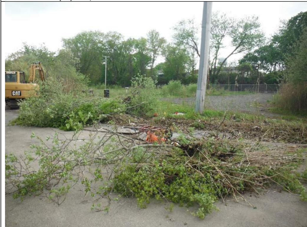
Photograph #26 – Cleared interior of the Site (between 212 and 234 West Main Street properties) (view looking southwest)
