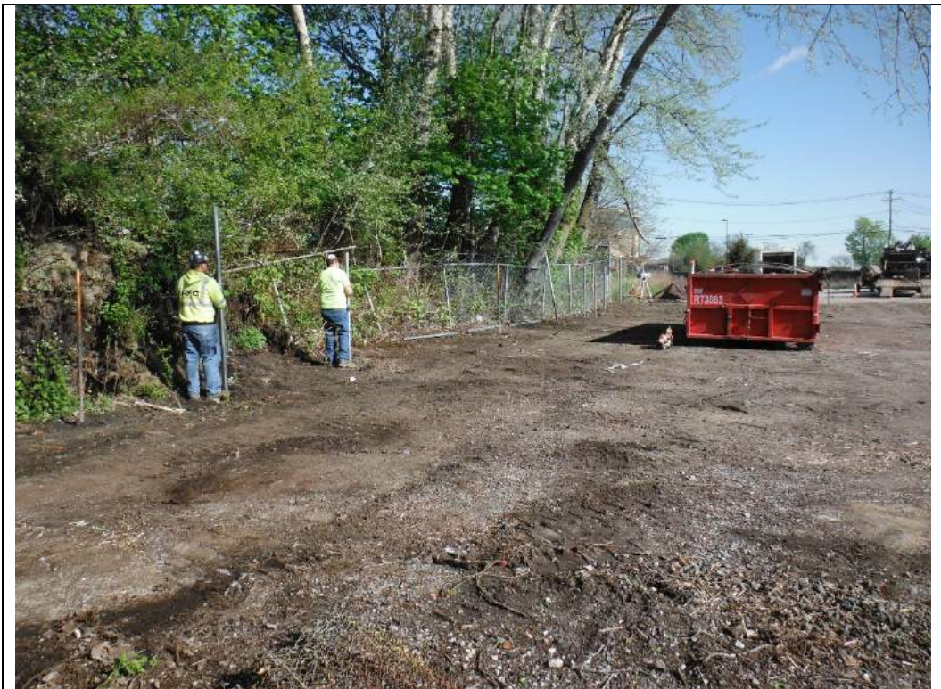
Photograph #13 – Setting posts along the western perimeter of the Site (view looking north)
