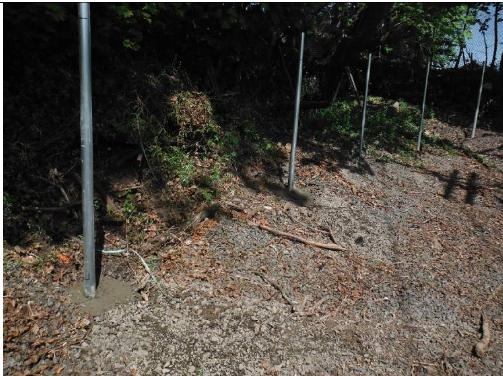
Photograph #16 – Installed fence posts along the western perimeter of the Site (view looking north)
