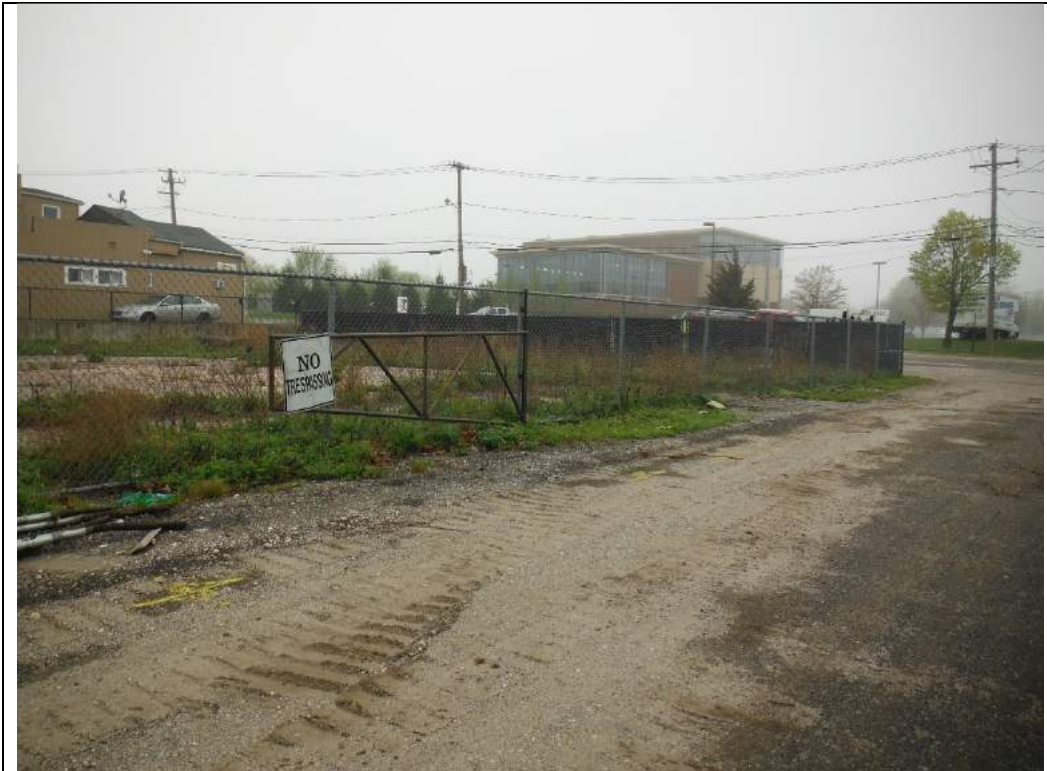
Photograph #3 – Existing gate and entrance across gravel driveway, prior to intrusive activities (view looking northwest)
