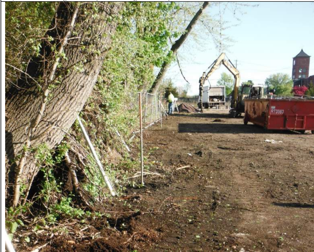
Photograph #12 – Excavation along western perimeter of the Site (view looking north)
