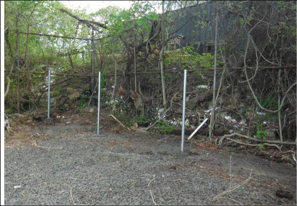
Photograph #17 – Installed fence posts along the western perimeter of the Site (view looking southwest)
