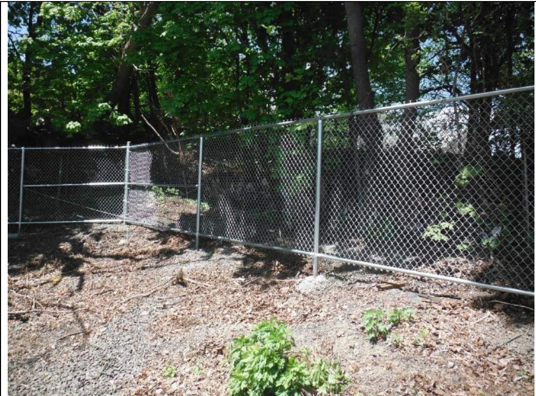
Photograph #19 – Completed fencing along western edge of the Site (view looking northwest)
