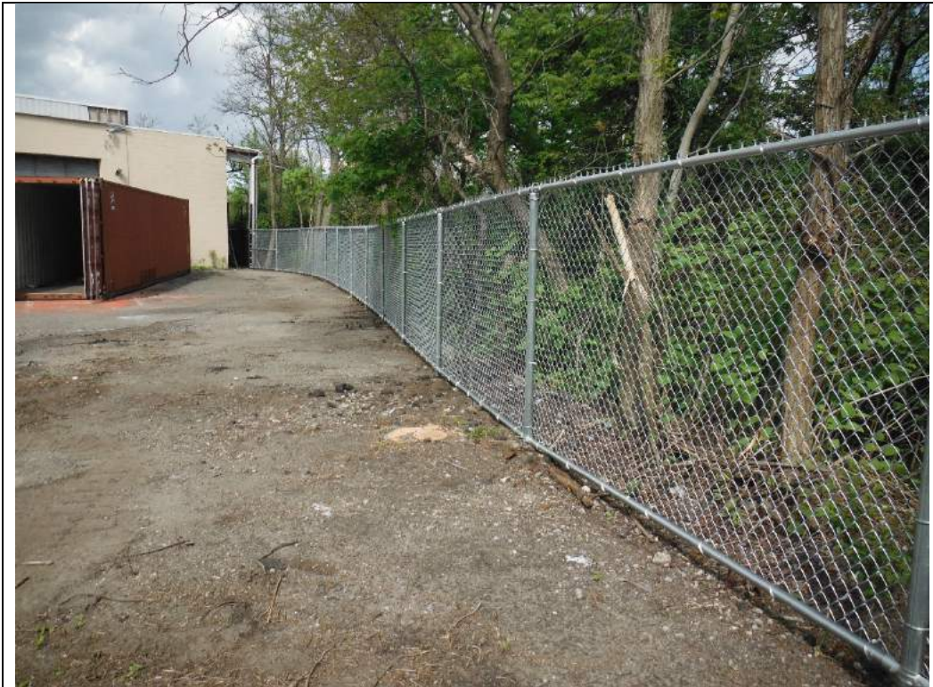
Photograph #21 – Completed fencing along the eastern perimeter of the 212 West Main Street property, adjacent to Patchogue River (view looking northeast)
