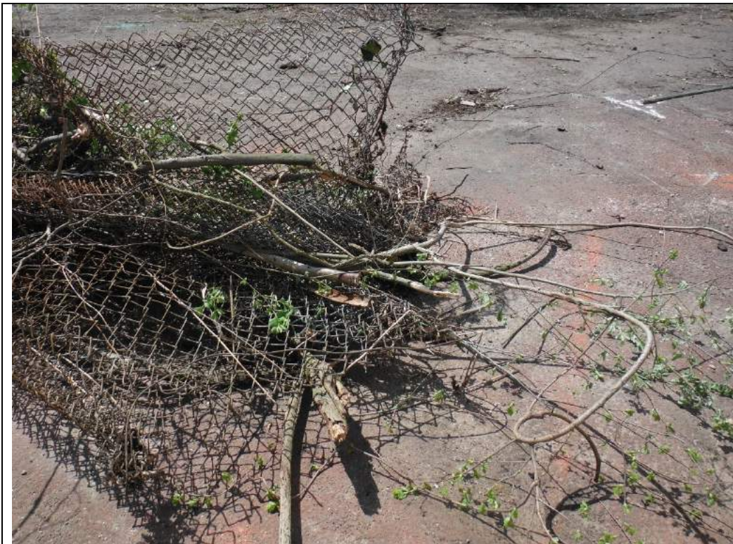
Photograph #25 – Removed fencing and vegetation from interior of the Site (between 212 and 234 West Main Street properties)
