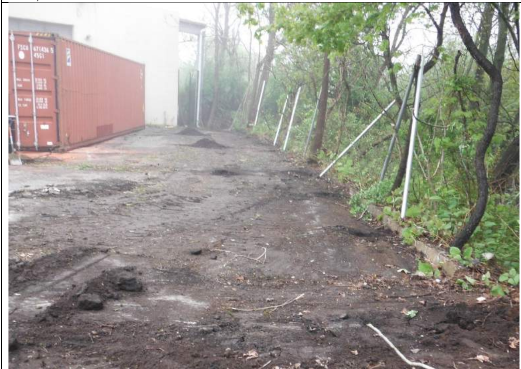
Photograph #10 – Removed fencing and posts and excavated post holes along east side of 212 West Main Street property, adjacent to Patchogue River (view looking northeast)
