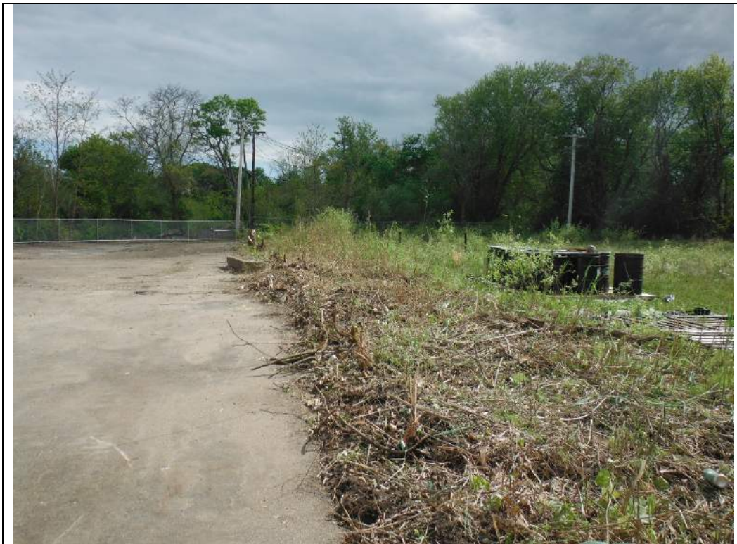
Photograph #27 – Cleared Site interior; work completed (view looking south)
