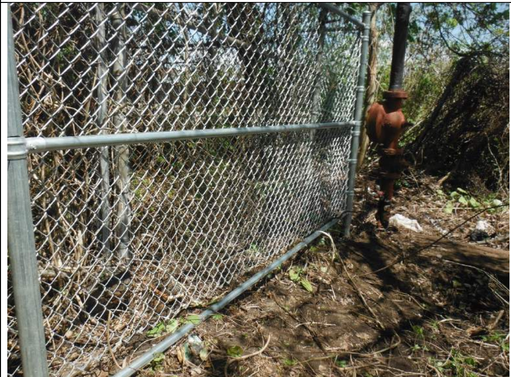
Photograph #20 – Completed fencing along western perimeter of the Site (view looking east)
