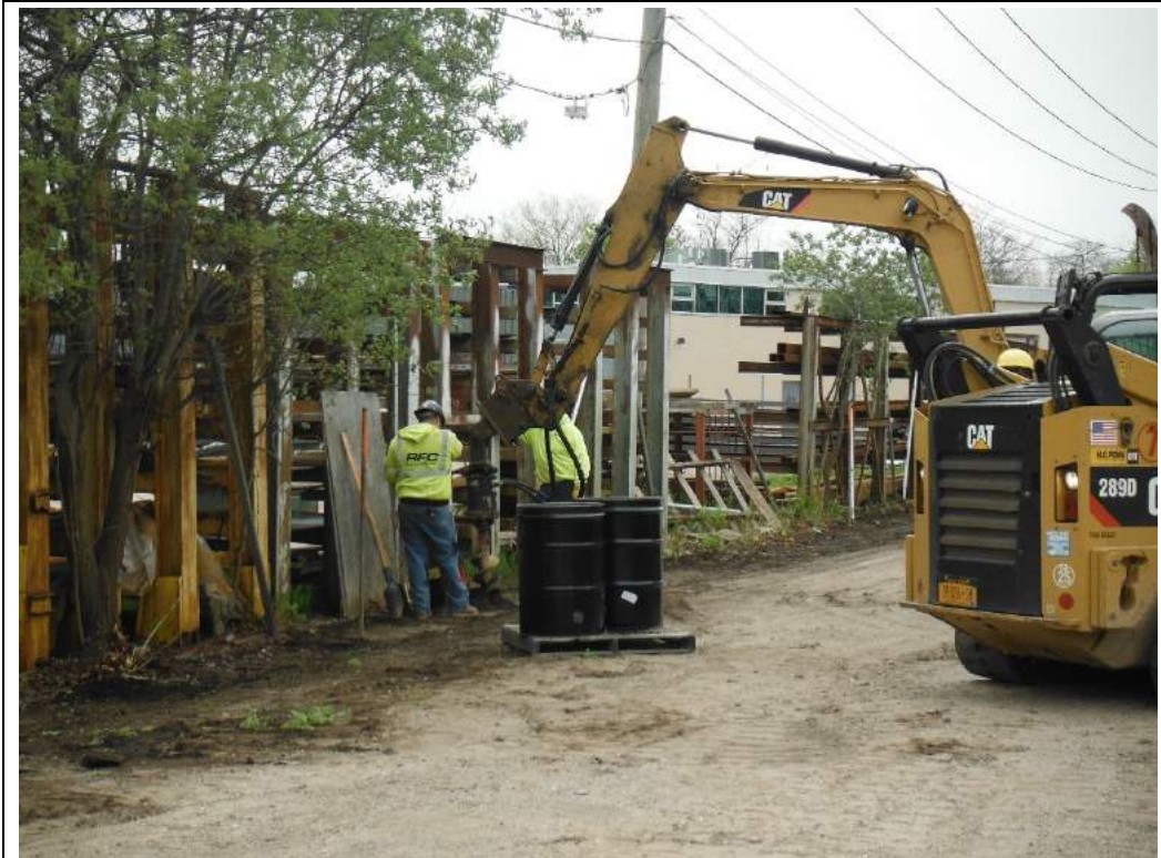
Photograph #5 – Contractors excavating fence post hole using backhoe mounted auger, depositing soil into 55-gallon drums, along eastern side of gravel driveway (opposite Site) (view looking southeast)
