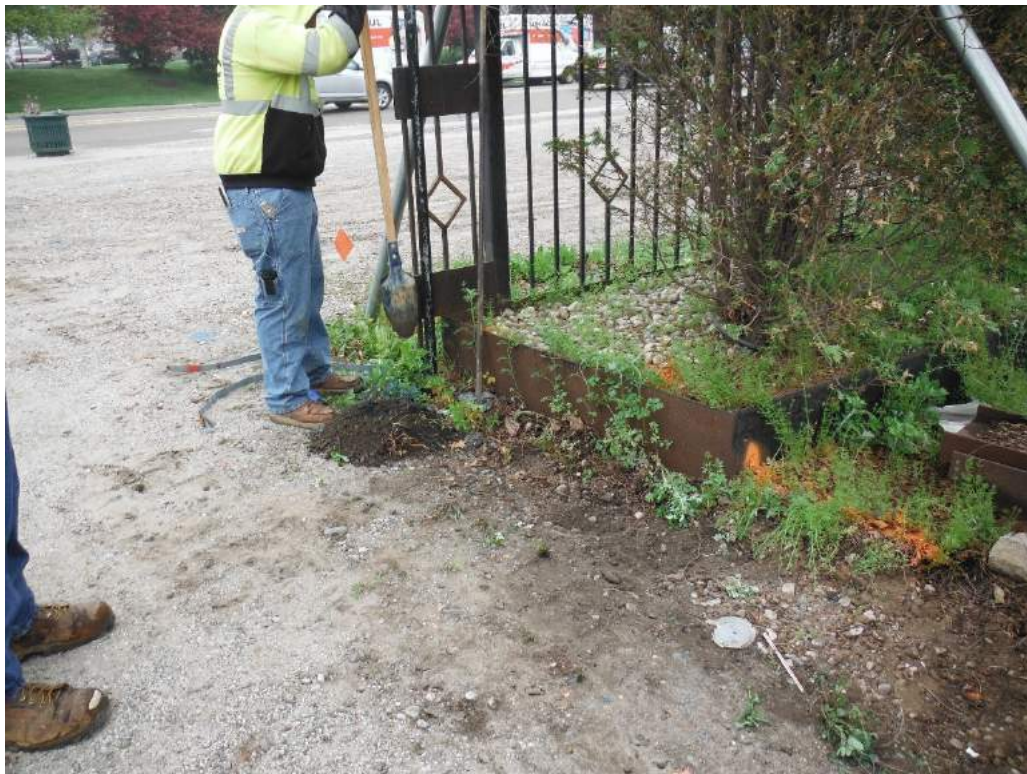
Photograph #4 – Manual post hole excavation at northeastern corner of site entrance (view looking north)
