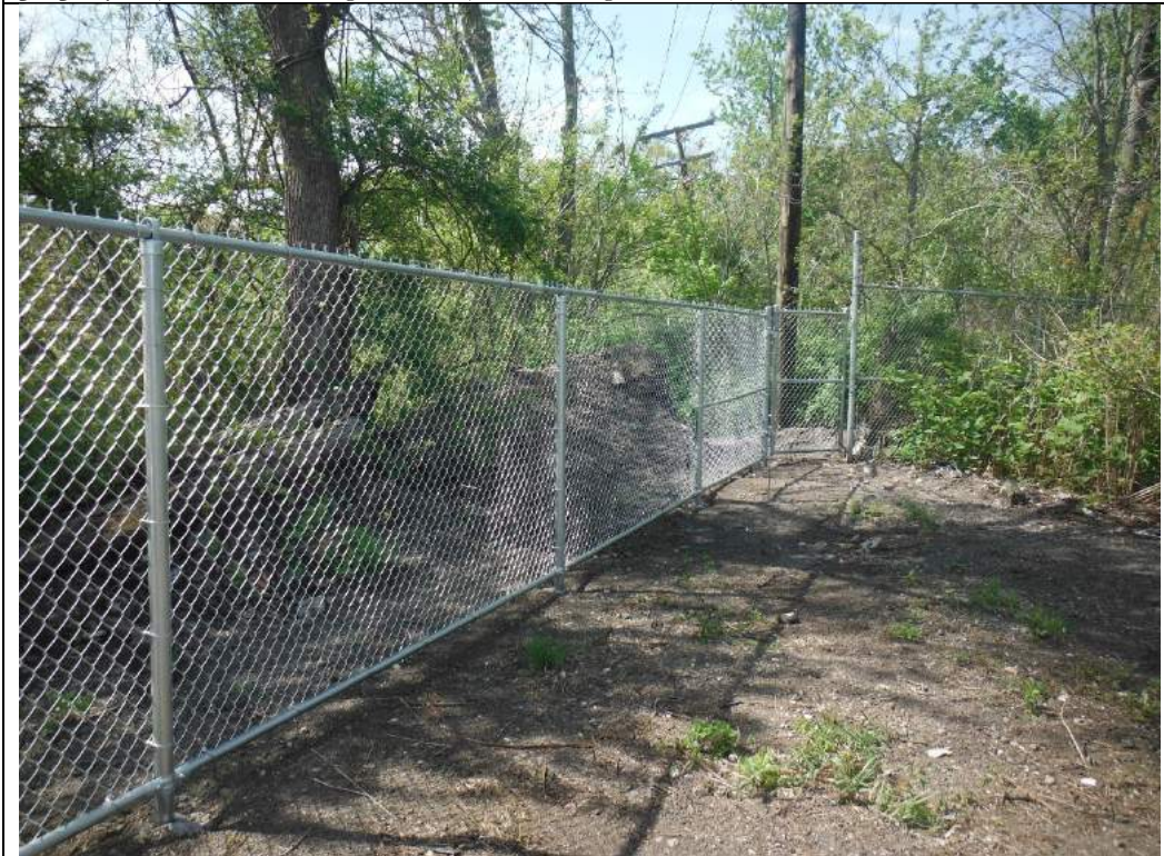
Photograph #22 – Completed fencing and gate along the eastern perimeter of the 212 West Main Street property, adjacent to Patchogue River (view looking southwest)
