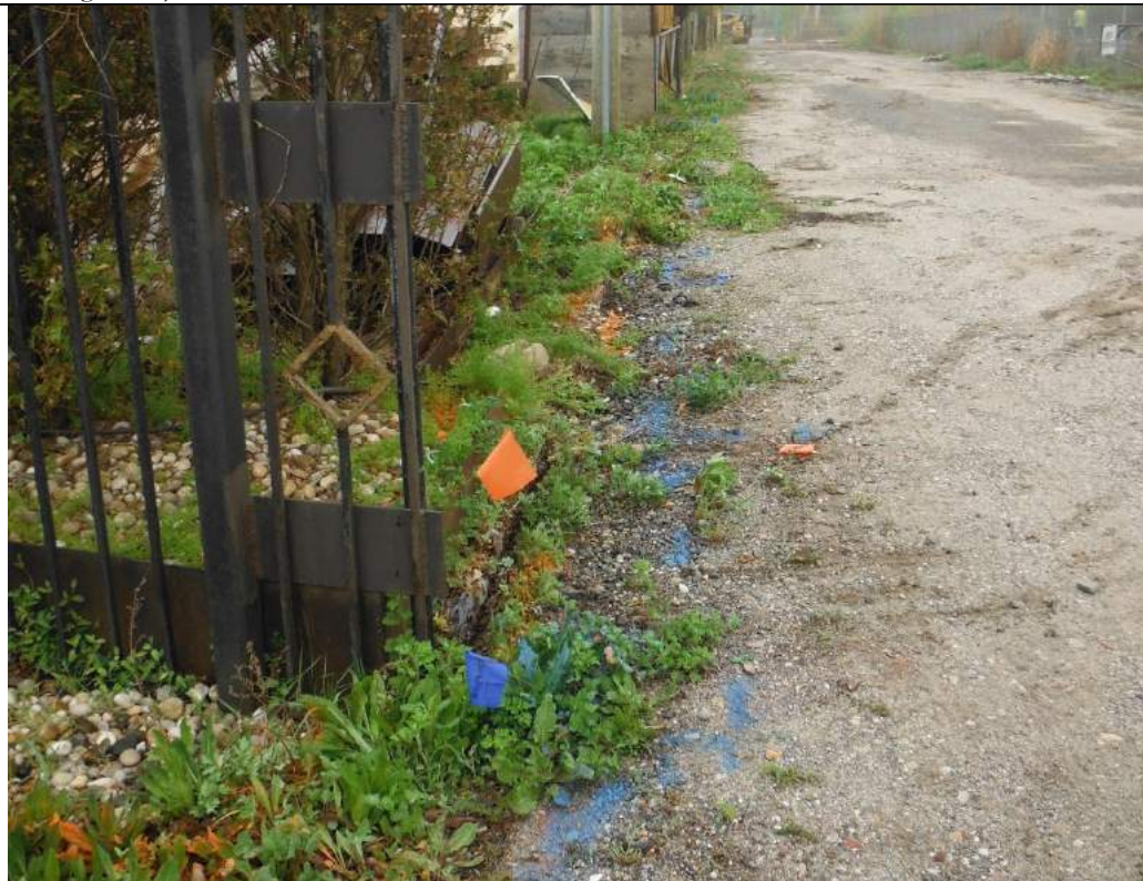
Photograph #2 – Utility mark-out along eastern side of driveway (opposite Site), prior to intrusive activities (view looking south)
