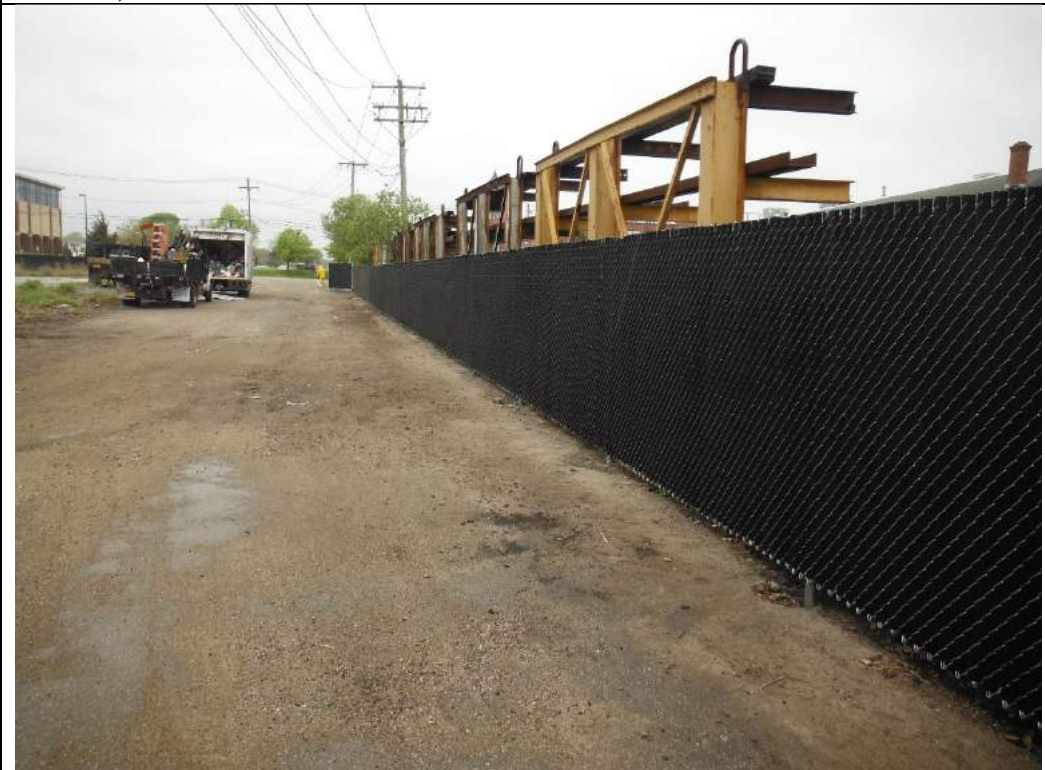
Photograph #18 – Completed fence (with privacy slats) on eastern edge of gravel driveway (view looking north)
