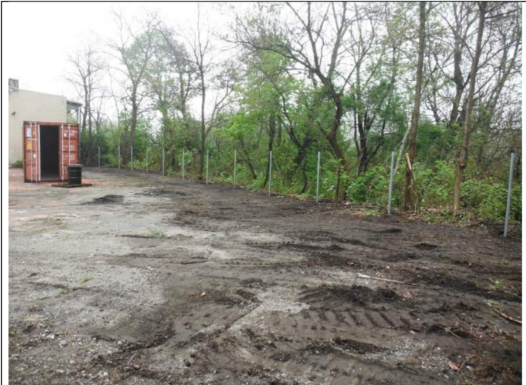
Photograph #11 – Installed fence posts along eastern side of 212 West Main Street property, adjacent to Patchogue River (view looking northeast)
