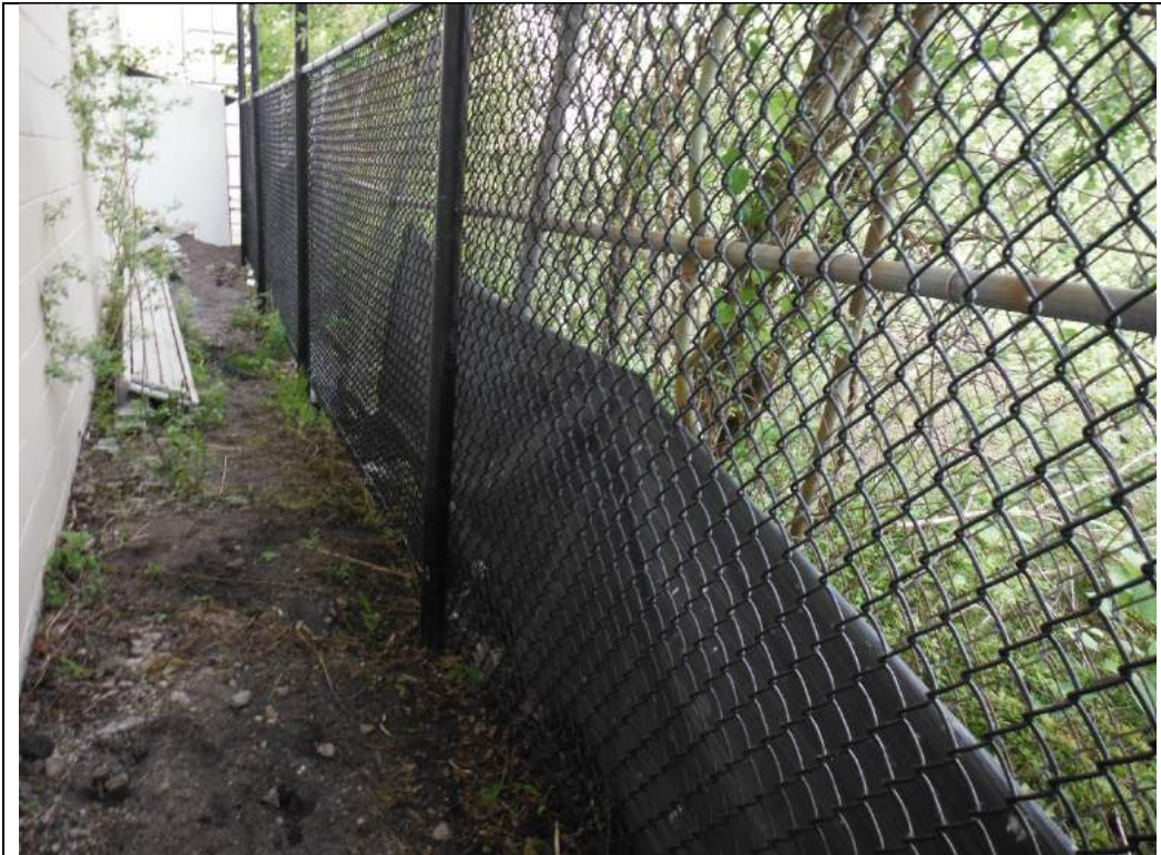
Photograph # 23 – New fence fabric installed on the eastern edge of the 212 West Main Street property, adjacent to building and Patchogue River (view looking northeast)
