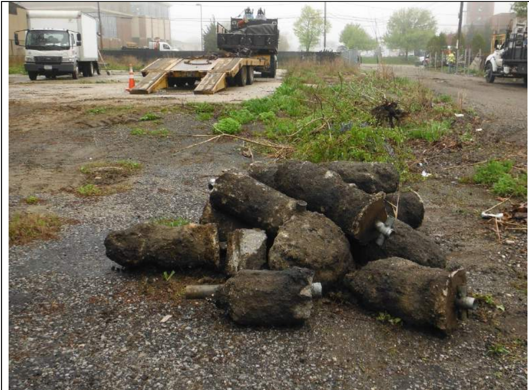
Photograph #9 – Removed fencing foundations from western side of gravel road (view looking north)
