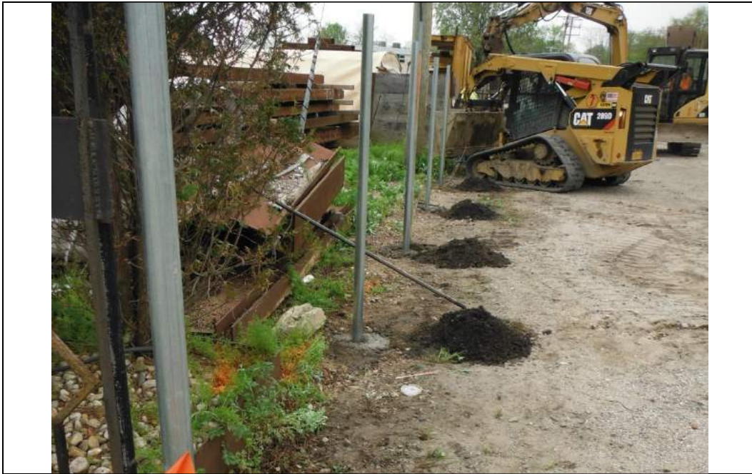
Photograph #7 – Contractor pouring concrete into an excavated fence post hole, excavated material directly next to the hole for inspection prior to containerizing in 55-gallon drums (view looking south)
