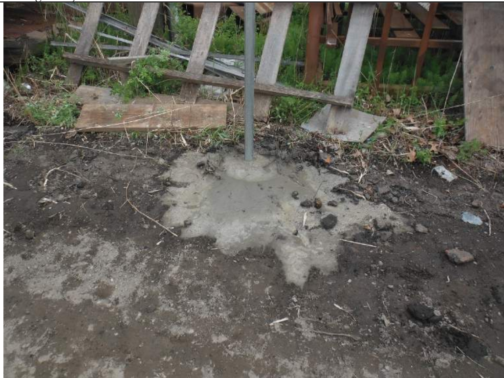
Photograph #8 – New concrete post footing along eastern edge of gravel driveway (view looking east)
