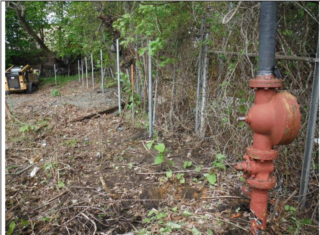
Photograph #15 – Installed fence posts along western perimeter of the Site (view looking west)
