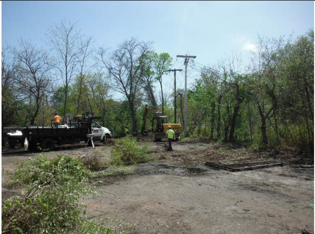
Photograph #24 – Clearing vegetation and existing fencing at grade from interior of the Site (212 West Main Street and 234 West Main Street properties) (view looking south)
