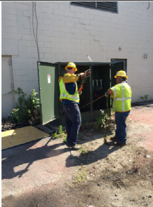
Photograph #7 – PSEG Long Island onsite to de-energize transformer to facilitation electric service installation.
