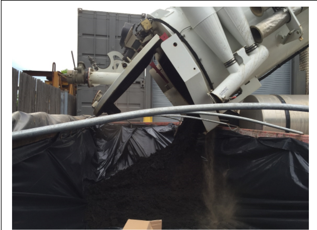
Photograph #5 – Transfer of wastes from the vacuum soil extraction unit into lined roll-off containers off-site disposal.
