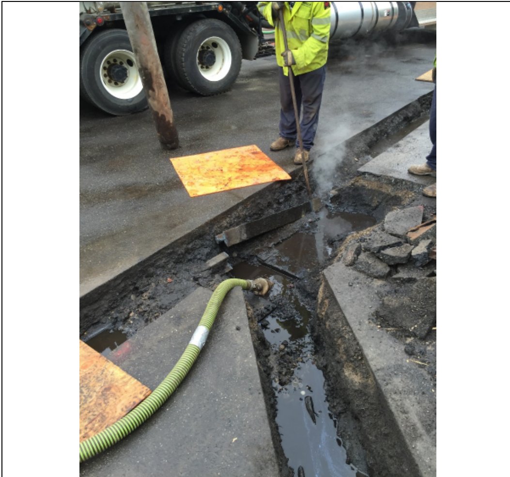
Photograph #8 – Removal of section of railroad track to facilitate electric service installation. Image notes dewatering activities.
