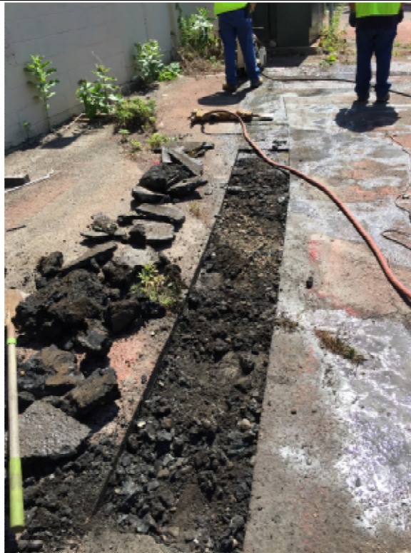
Photograph #3 – Saw cutting and removal asphalt along trench alignment south of off-site building.
