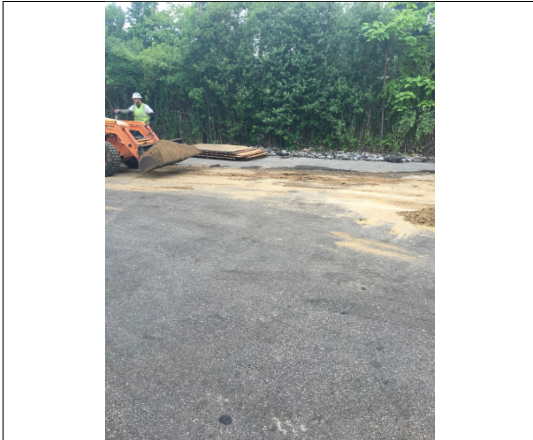
Photograph #10 – Backfilling activities.
