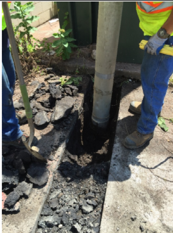
Photograph #4 – Vacuum extraction of soils to 30-inches bgs for underground electric service installation.
