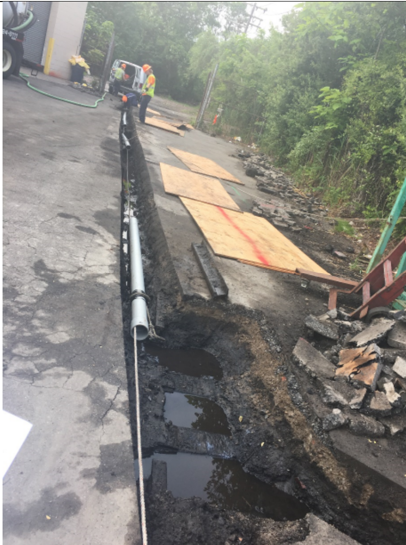
Photograph #9 – PSEG Long Island installation of underground electric service. Schedule 80 PVC used where electric line had potential to come into contact with metal debris (railroad track), or trench depth did not meet prescribed depth of 30-inches bgs.
