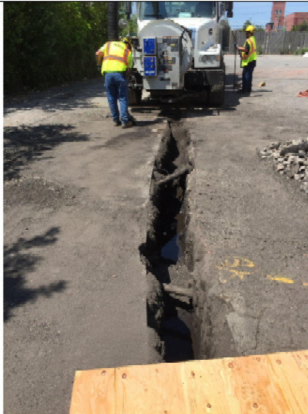
Photograph #6 – Vacuum extraction of soils underground electric service installation. Image notes buried utilities and abandoned railroad tracks.
